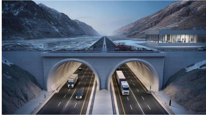
Figure 4.3: China's 22.13 km Tianshan Shengli Tunnel, Xinjiang
